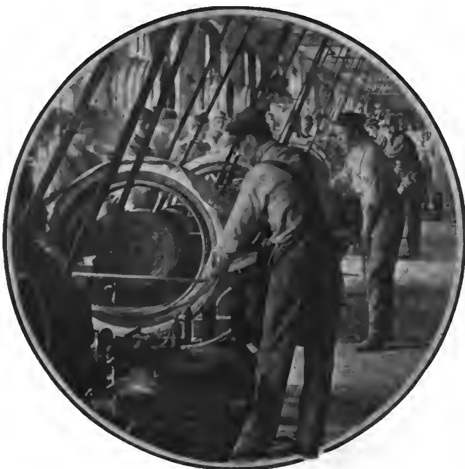
After cleaning, the tread is applied as shown
